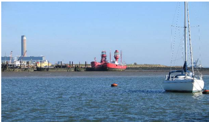
Looking backwards to Kings North power station on the Medway
